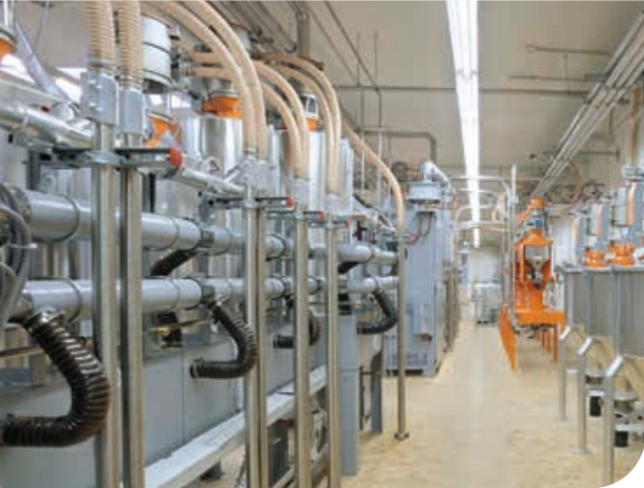
Suction & transport hoses used for filling granule dryers along with temperature-proof hoses for transporting the air for the dryer itself
